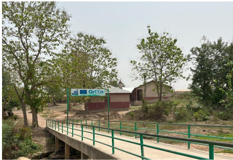
Figure 2: Climate resilient infrastructure (bridge), Ashanti, February 2025 (Altai Consulting)
