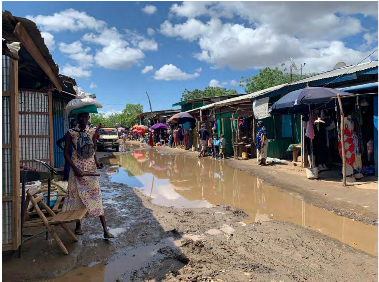
Fig. 32: Flooded Section of Ethiopian Market Street (UN-Habitat, 2022)
