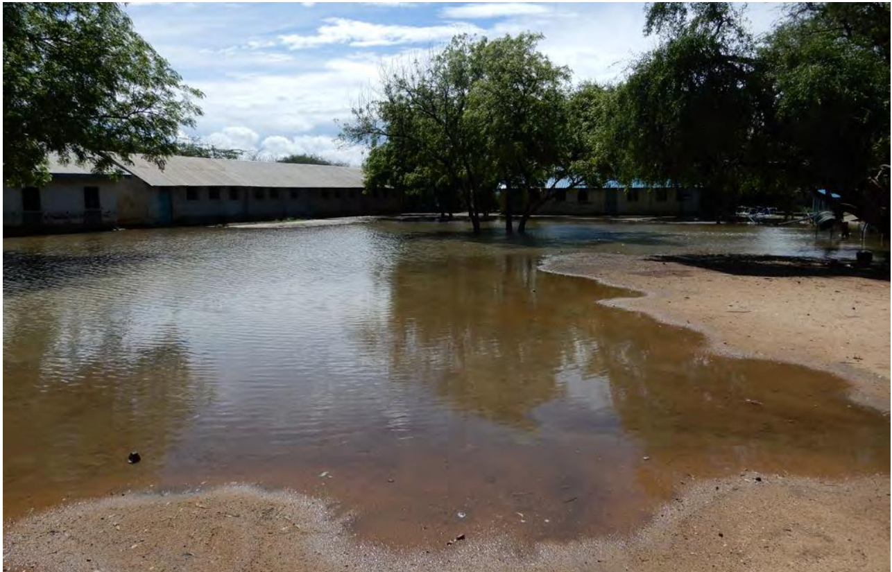
Fig. 31: Flooded School Compound at Gilo ECD (UN-Habitat, 2023)
