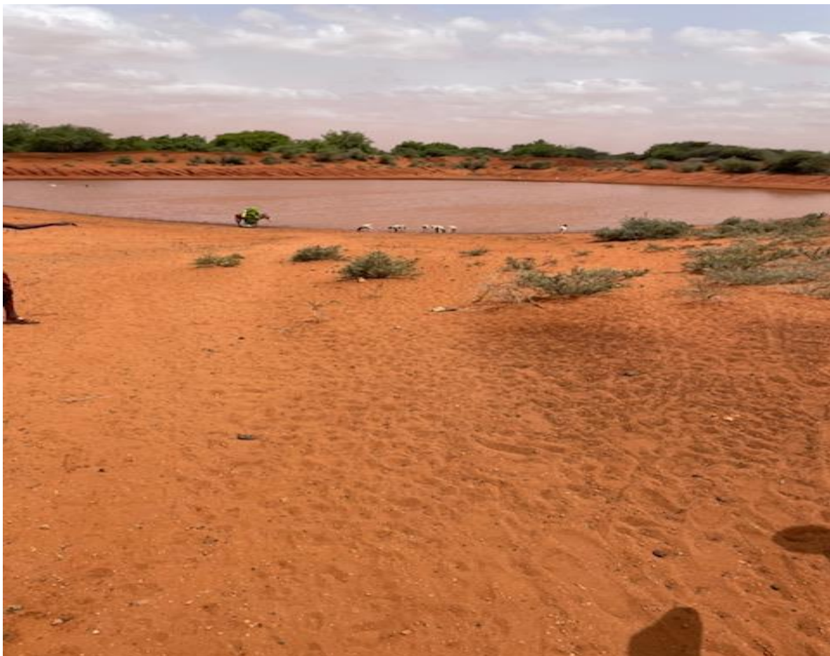
Figure 7: Dam built in the 1950s in Duruqsi, Somaliland
