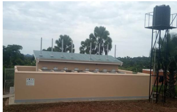
Picture 16: Eight-stance VIP latrine at Lasanga Health Centre III, Koboko Municipality
